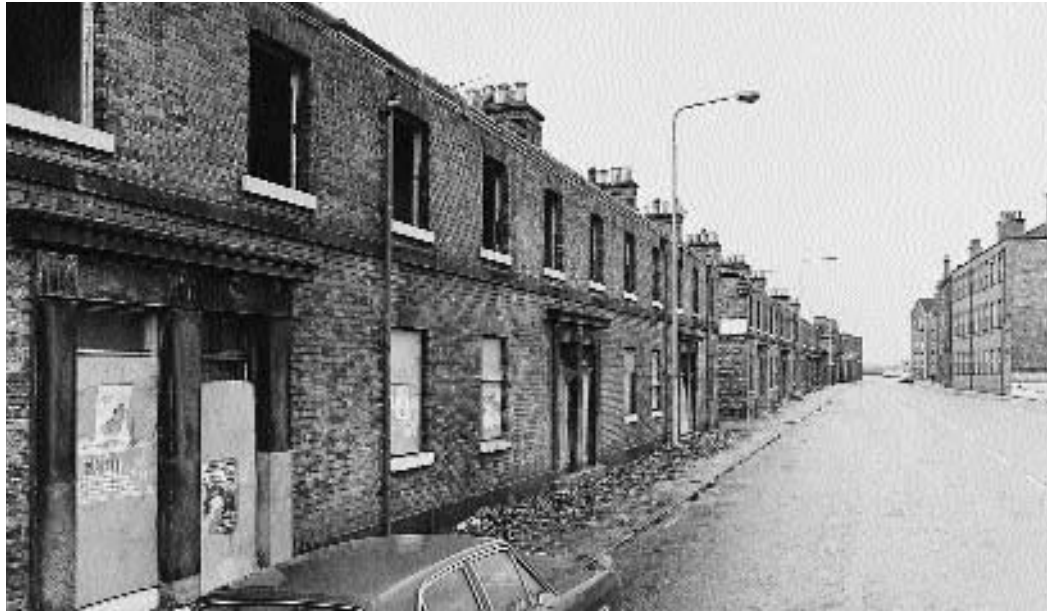
Figure 5.22 Railway Cottages, Derby. Before rehabilitation.
